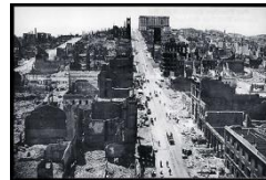
1906: San Francisco Earthquake
