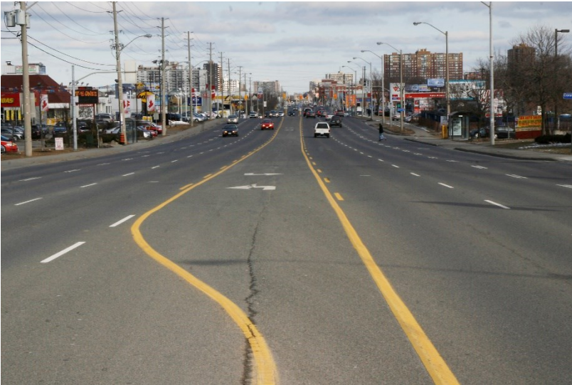
Eglinton Avenue Toronto (Now)
