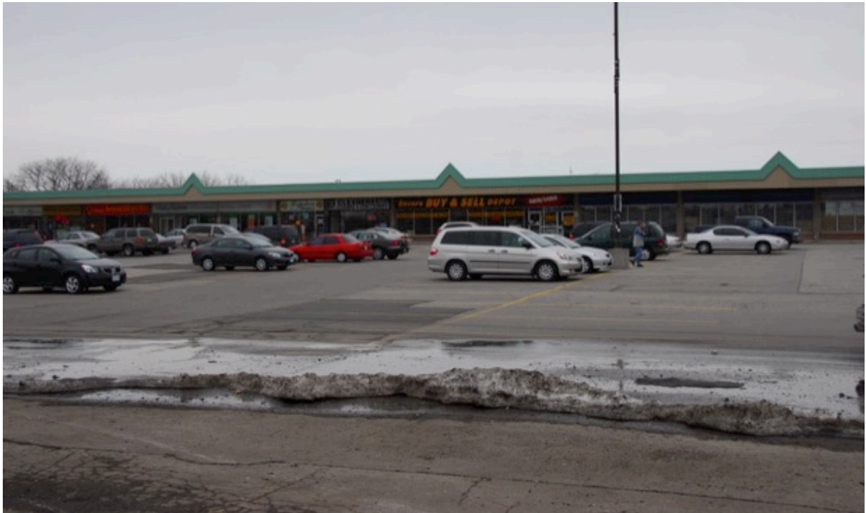
Figure 7 Retail sites along Scarborough arterial roads are prime redevelopment sites
