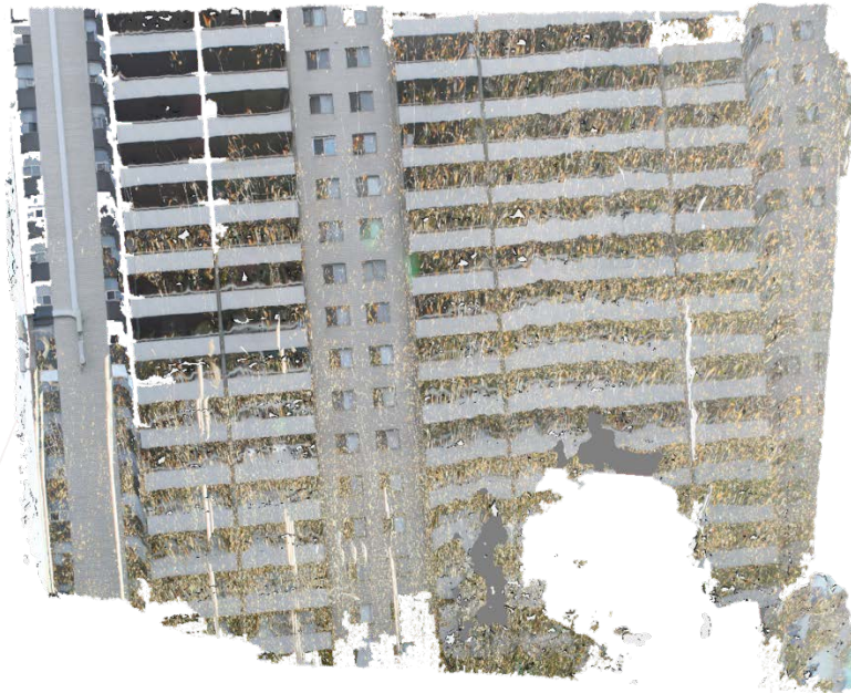
Figure 24. Photogrammetry model of apartment building adjoining park
