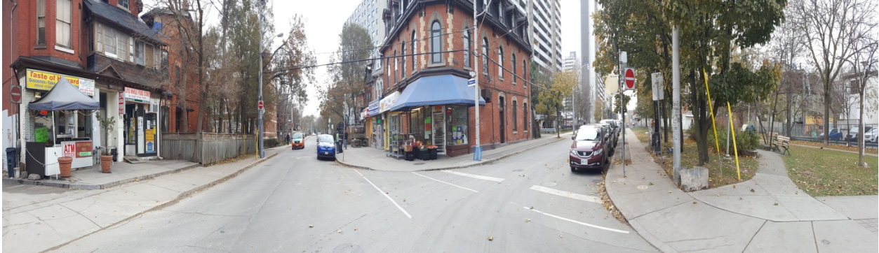
Figure 17. Panoramic view of Howard Street and Bleecker Street intersection, St. James Town
